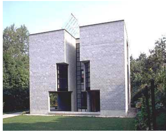
Figure 9 Botta's building in Pregassona (CH).
